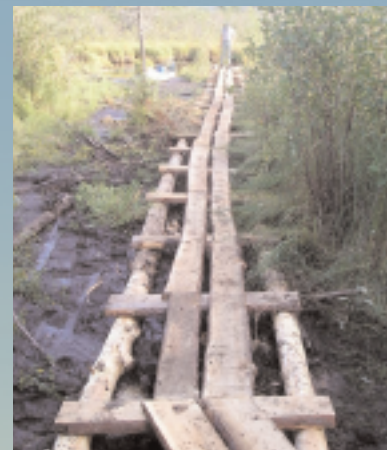
Before and after photos of a boardwalk installed in 2004 to prevent resource damage from occurring on the Trident Lake to Frog Lake portage. A year of vegetation growth and weathering will naturalize this feature.
